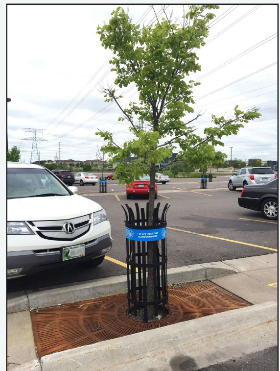
Tree planted in tree trench; note the curb and tree cage used to protect trees from car damage.
