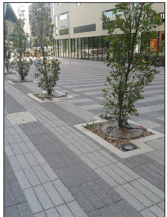
Trees planted in an urban area. Permeable pavement is used throughout to allow infiltrating runoff to reach the roots.
