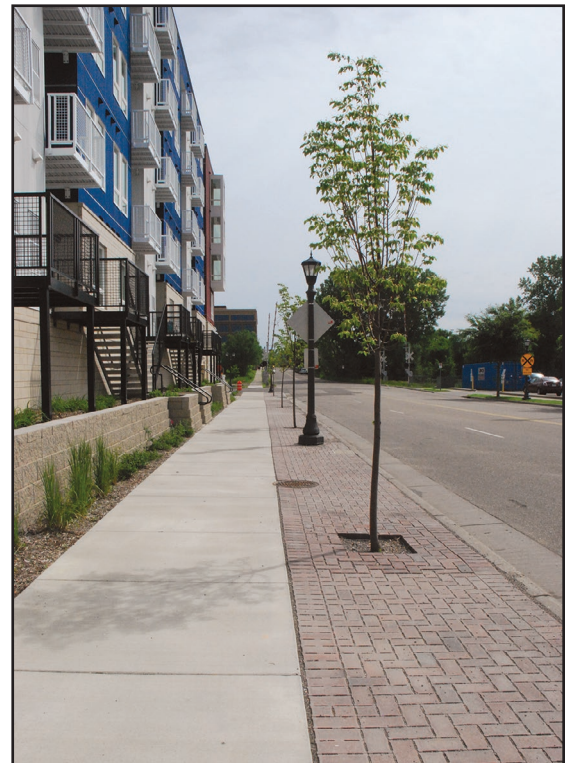
Young trees planted in urban environment. A portion of the sidewalk is permeable pavement to allow rainwater to seep into root areas.
