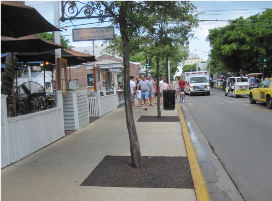
Permeable pavements increase infiltration, helping trees receive oxygenated water and reduce stormwater runoff. When used in conjunction with other engineered systems designed to grow big trees and manage stormwater, permeable pavements can boost the infiltration rate and amount of runoff entering the system. Photo courtesy of Davey Resource Group.
